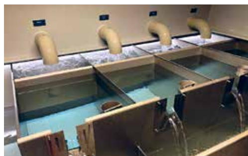
Source_ drinking water: Groundwater from the Luxembourg Sandstone make the region self- sufficient in drinking water.
