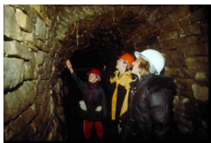
Underground in Carr's Mine
