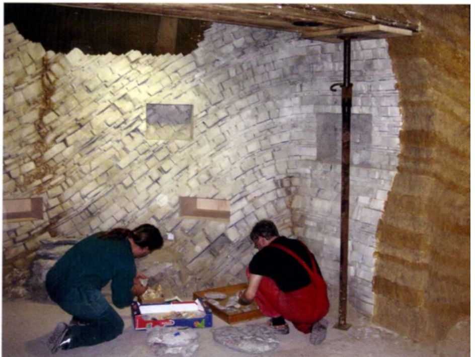
TERRA.vita information centre: The "Upper Cretaceous quarry" in construction
